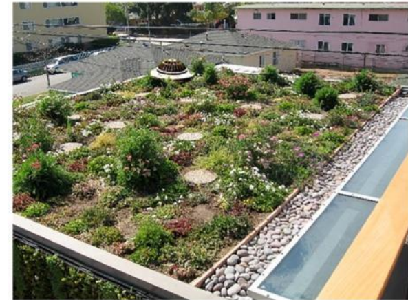
Bioretention system with rock pitching and overflow pit.
