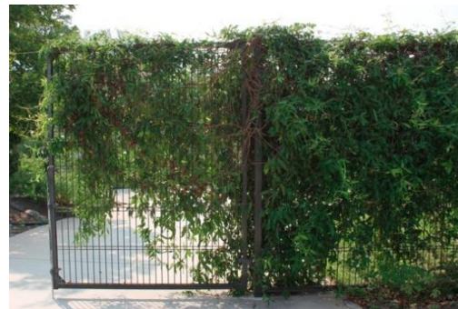
Figure 42 - New high fence
