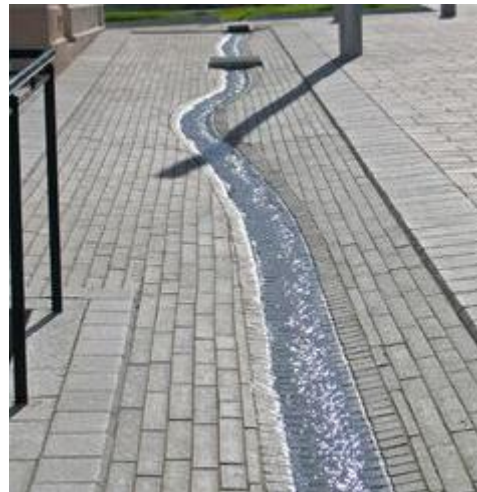
Figure 55 - Urban surface water channel
