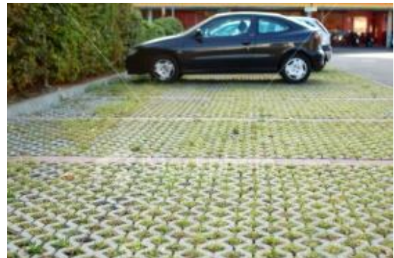
Figure 45 - New pavement for the parking lot
